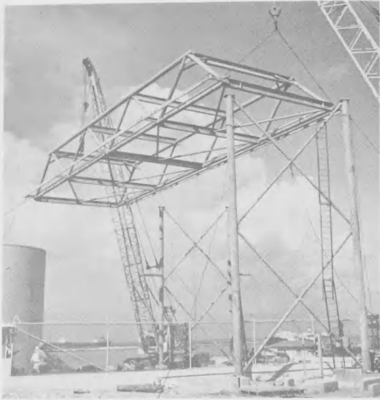
THE FOURTEEN-ton truss section of Lago's new pipe bridge was erected by the contractor March 19 with the aid of Lago's two heavy-duty cranes. Forty-foot columns support the section. E SECCION di aguante di diez-cuatro ton na e brug nobo di tubo na Lago a worde erigi door di e contratista Maart 19 cu ayudo di e dos gruanan pisá di Lago. Columnanan di cuarenta pia ta wanta e seccion.
